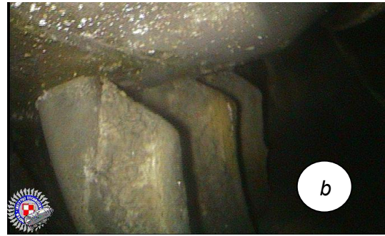
Figure 9b. Turbine vanes operated in the heavy dust conditions [4]
